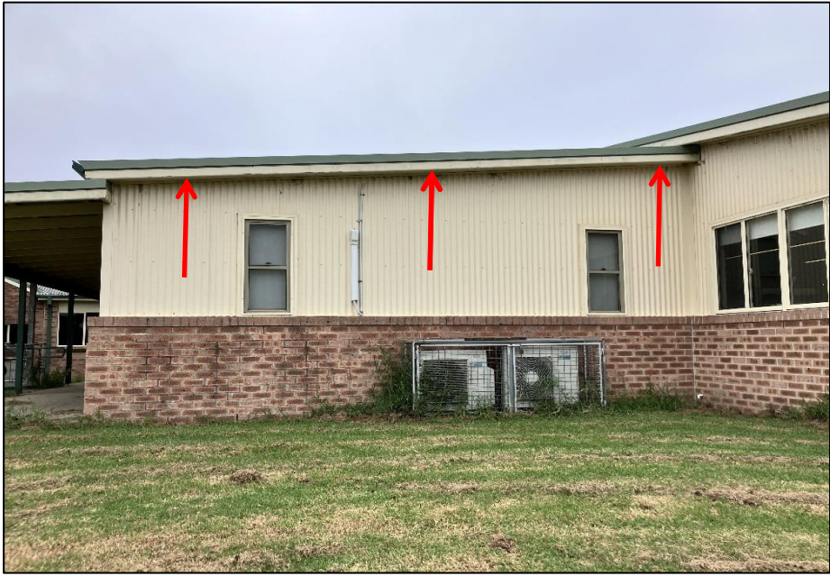
Photograph 3: B00V, exterior, western façade, north end, eave lining, no asbestos detected by analysis.
