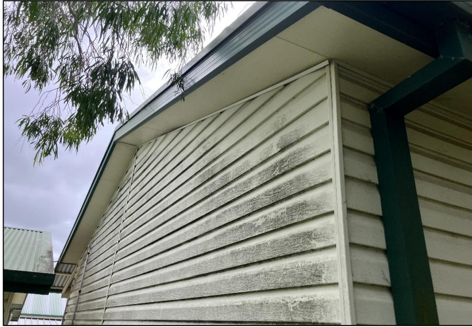
Photograph 1: B00S, exterior, eave linings, fibre cement sheeting, no asbestos detected by analysis.
