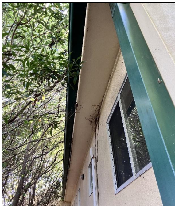
Photograph 3: B00W, exterior, northern façade, eave lining, fibre cement sheeting, no asbestos detected by analysis.
