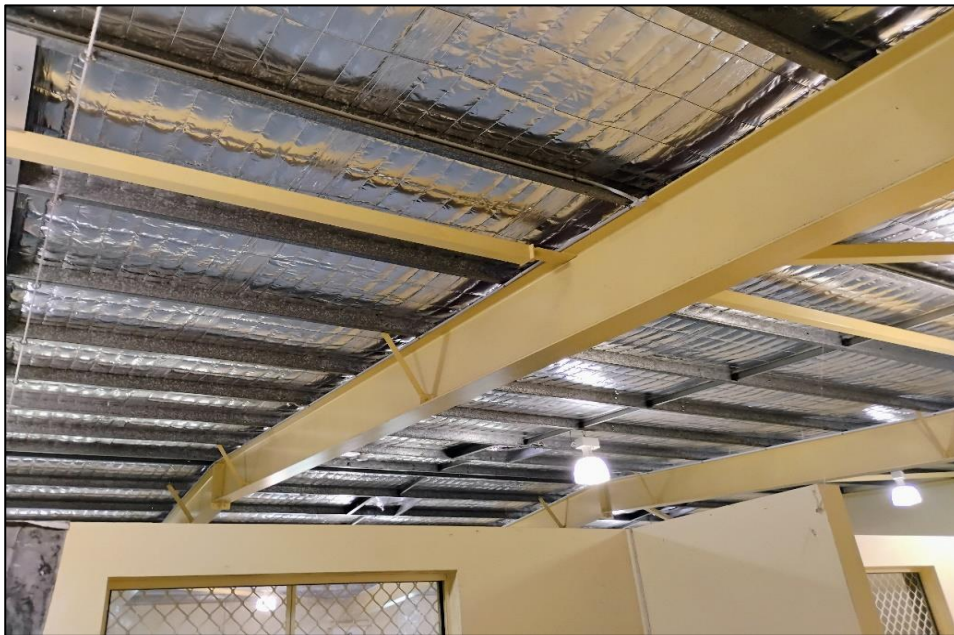
Photograph 5: B00I, interior, roof framework, steel beam, pale yellow paint.
