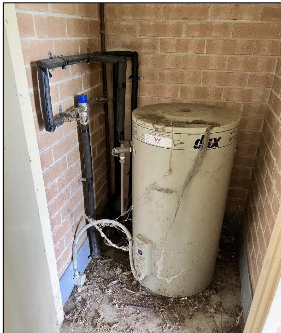
Photograph 10: B00A, AR0018, Dux hot water unit (circa 1998), insulation, SMF (suspected).
