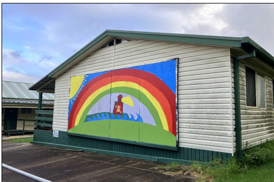
Photograph 2: B00T, exterior, mural, fibre cement sheeting, no asbestos detected by analysis.
