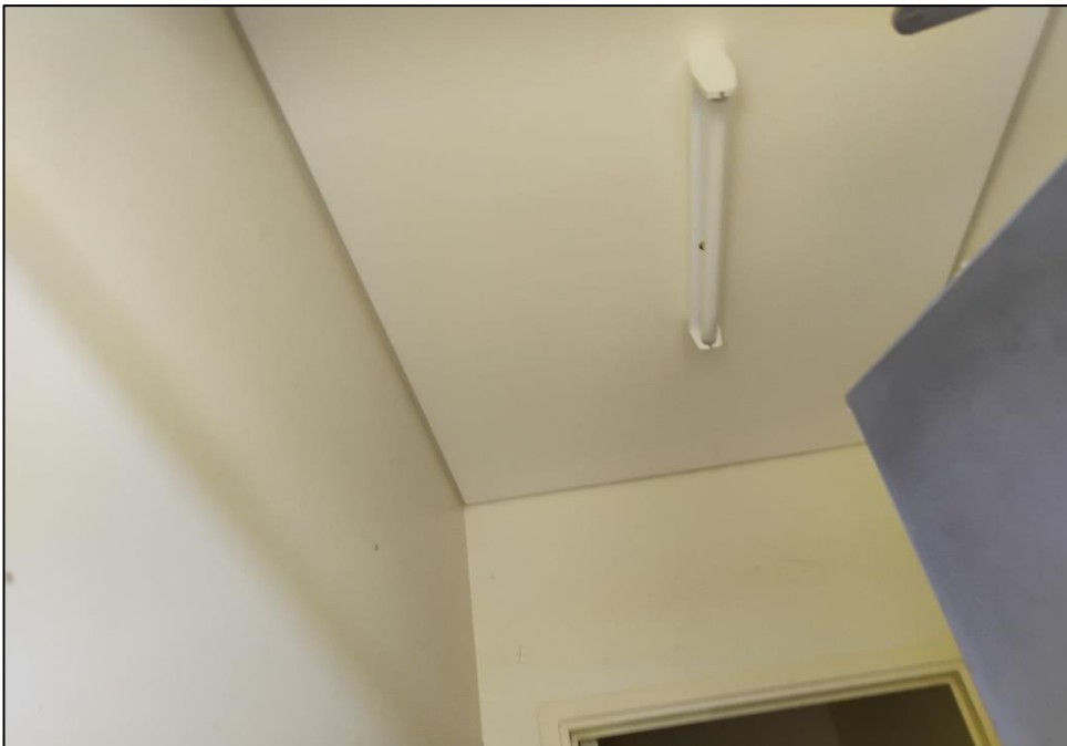
Photograph 6: B00E, interior, ER0021, linings generally, fibre cement sheeting, no asbestos detected by analysis.
