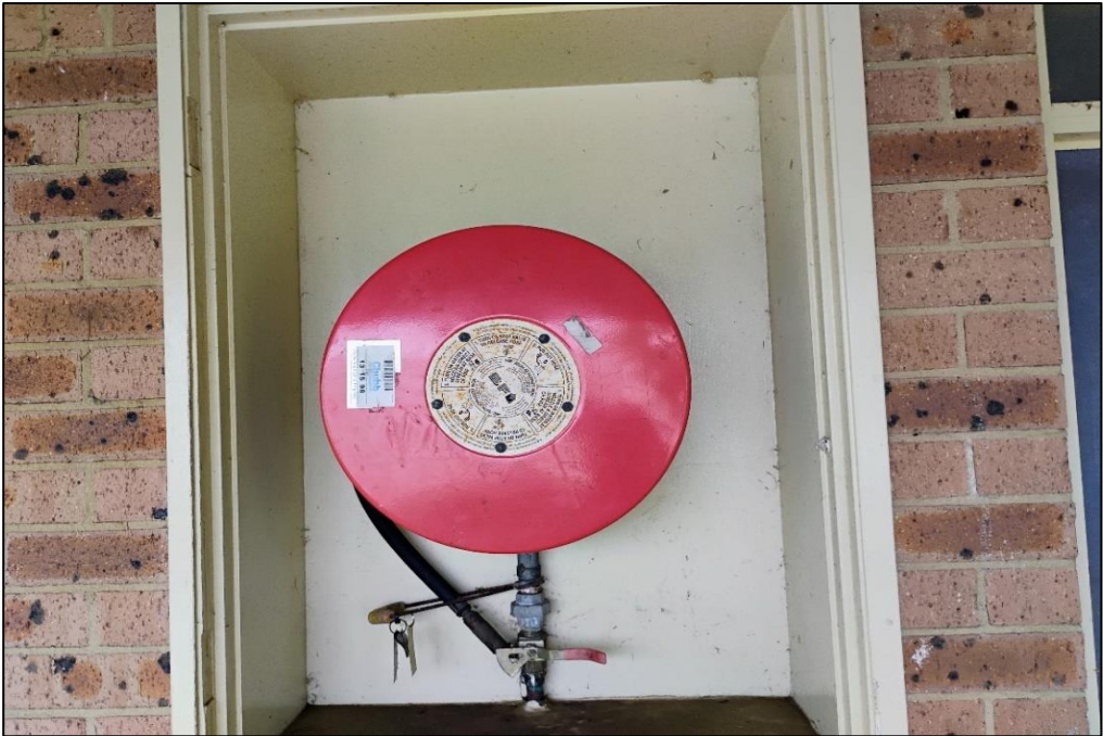
Photograph 5: B00D, exterior , west façade, fire hose recess wall, fibre cement sheeting, no asbestos detected by analysis.
