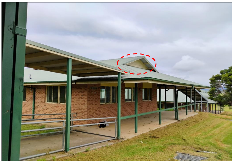
Photograph 1: B00D, exterior, north and south façade, gables, weatherboard linings, suspected non-asbestos.
