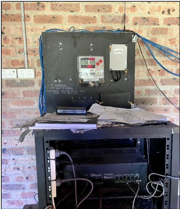
Photograph 8: B00W, WR0015, electrical panel, backing board, suspected non-asbestos.
