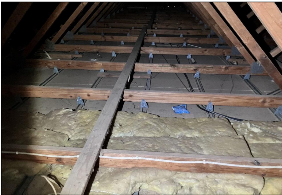
Photograph 8: B00C, rooms and areas in general, ceiling cavity, top of ceiling, insulation, SMF identified visually.
