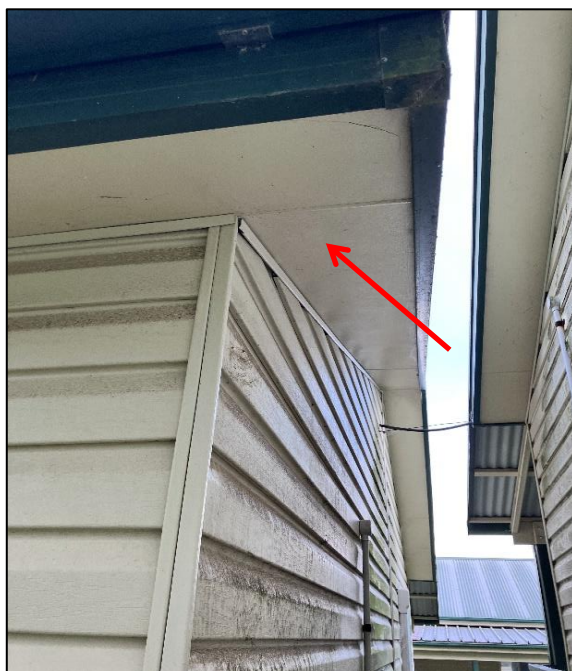
Photograph 1: B00T, exterior, eave linings, fibre cement sheeting, no asbestos detected by analysis.
