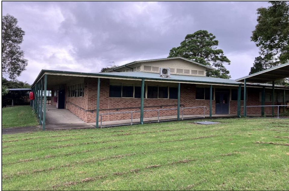
Photograph 11: B00B, exterior, roof, air-conditioning unit(s), unidentified, inaccessible.
