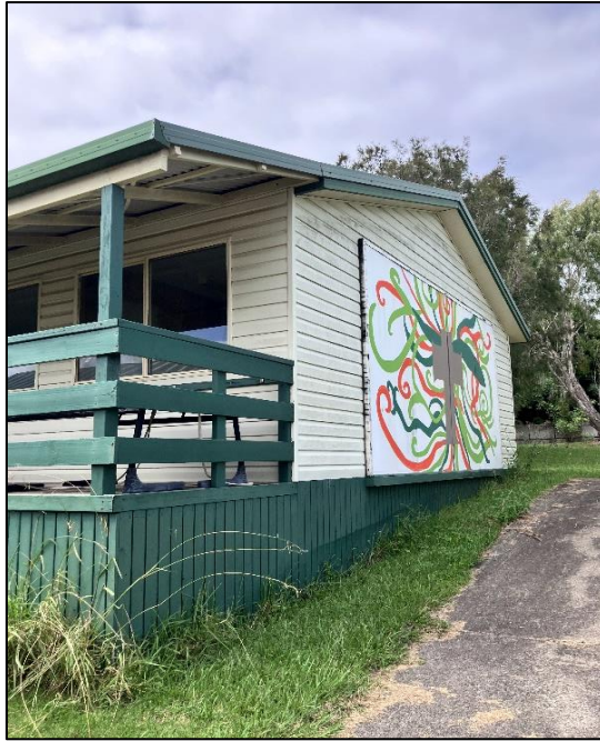
Photograph 3: B00R, exterior, subfloor area, materials in general, inaccessible.
