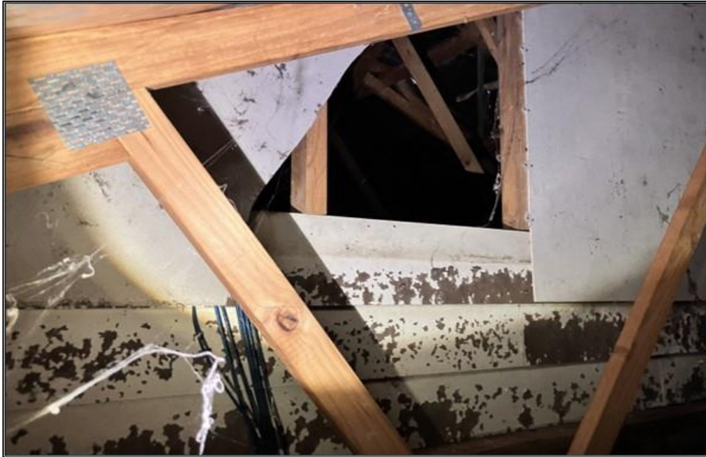
Photograph 7: B00P, ceiling cavity, bulkhead, fibre cement sheeting, no asbestos detected by analysis.
