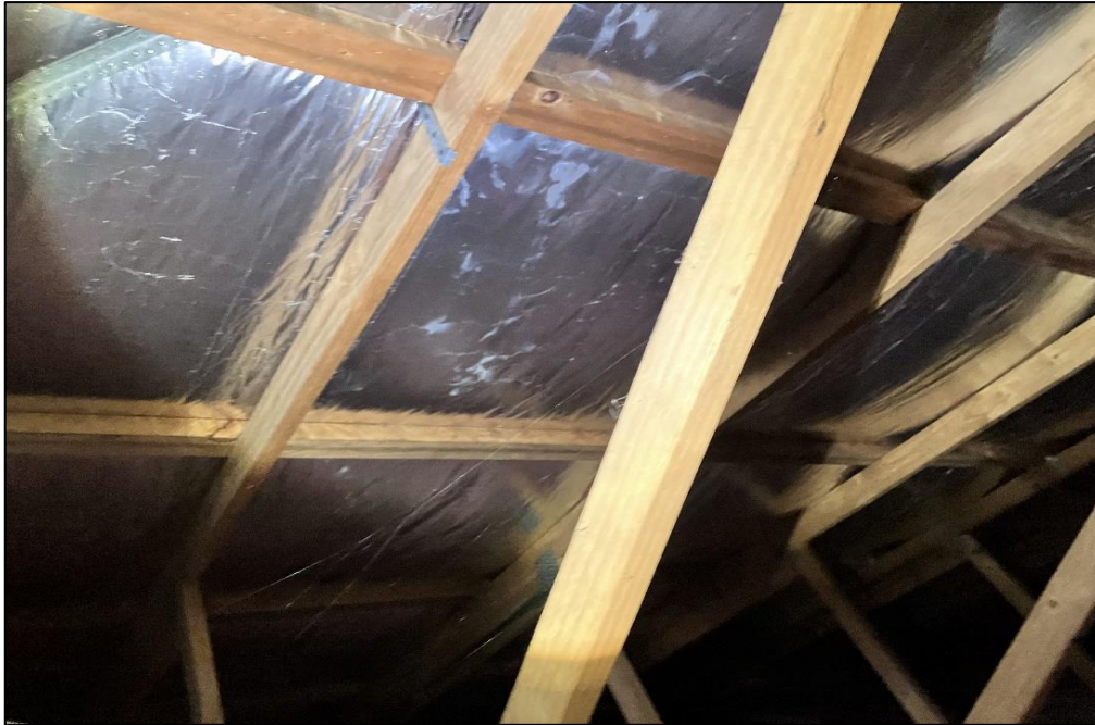
Photograph 9: B00P, rooms and areas in general, ceiling cavity, underside of roof, insulation, SMF identified visually.
