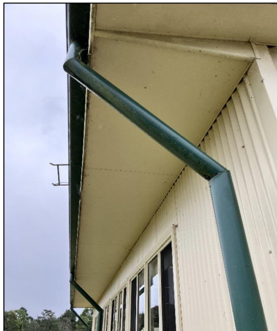
Photograph 2: B00V, exterior, western façade, centre, eave lining, no asbestos detected by analysis.
