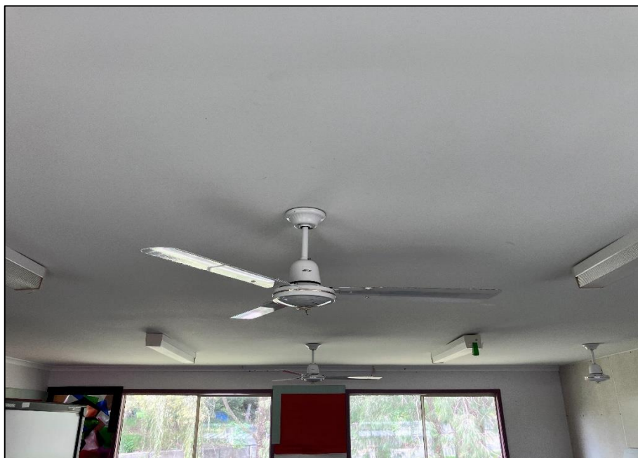
Photograph 7: B00R, rooms and areas in general, ceiling fans, internal components, nil PCB (suspected).
