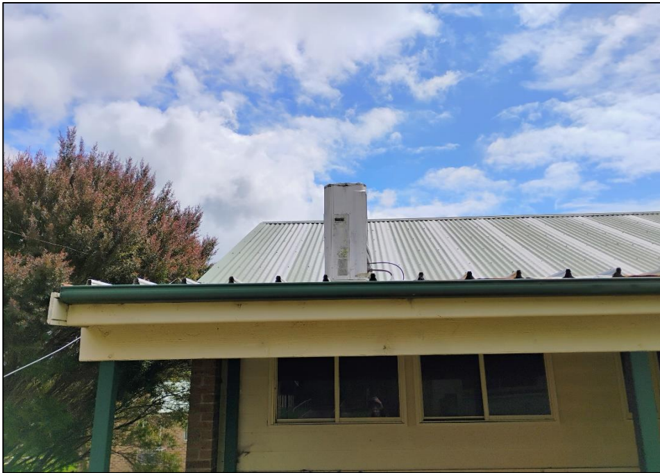
Photograph 9: B00Q, exterior,QR004, roof, air conditioning unit, R410A, nil ODS identified.
