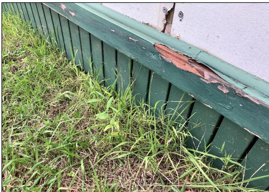
Photograph 5: B00R, exterior, southern facade timberwork, green paint.
