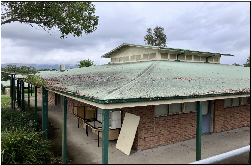
Photograph 1: B00B, exterior, upper level, walls, weatherboard linings, suspected non-asbestos.
