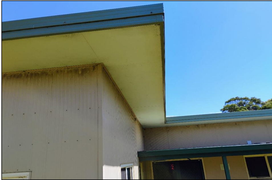
Photograph 1: B00H, exterior, southeastern façade, eave lining, fibre cement sheeting, no asbestos detected by analysis.
