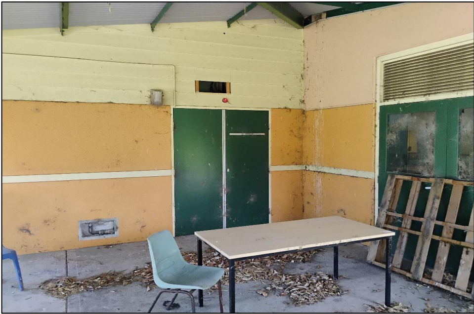
Photograph 1: B00I, exterior, northern façade, weatherboard headlining, fibre cement product, no asbestos detected by analysis.
