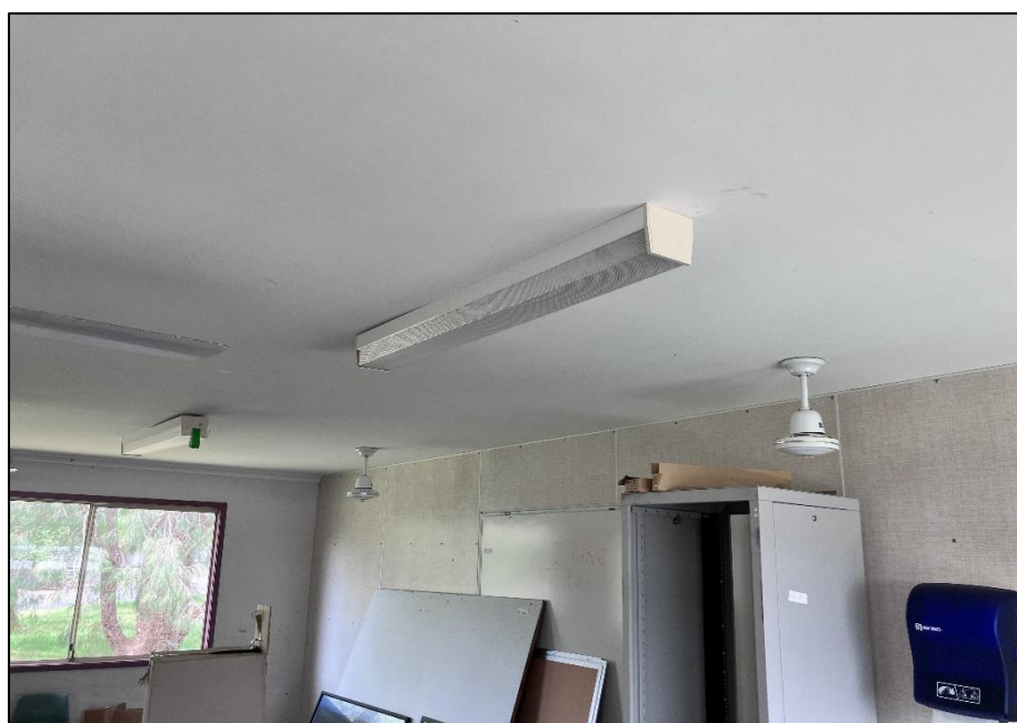
Photograph 6: B00R, rooms and areas in general, fluorescent light fittings, internal components, nil PCB (suspected).
