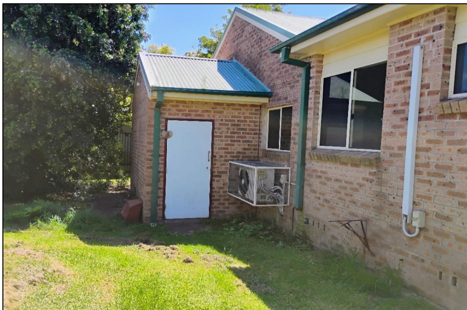
Photograph 10: B00W, WR0015, fire door, insulation, suspected non-asbestos.
