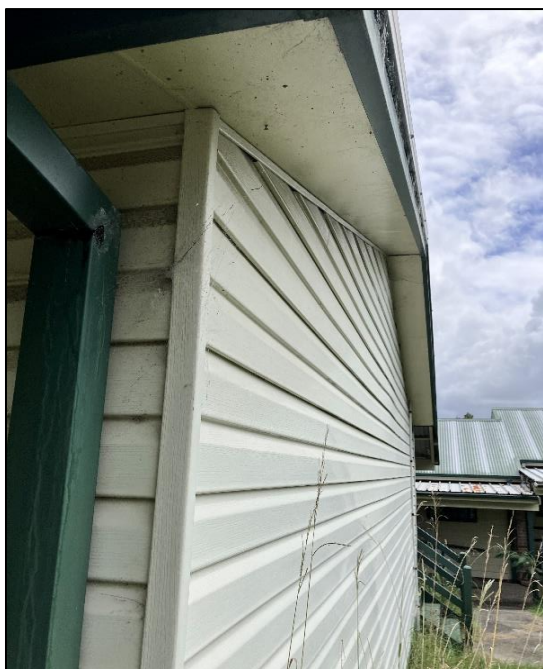
Photograph 1: B00R, exterior, eave linings, fibre cement sheeting, no asbestos detected by analysis.
