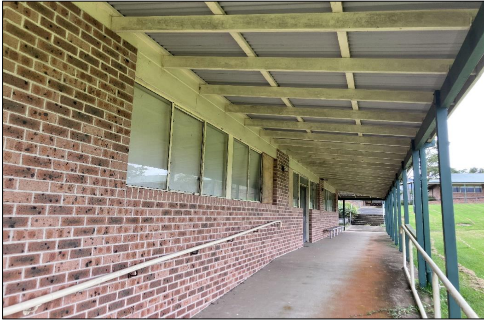
Photograph 3: B00A, exterior, lower level, walls generally, weatherboard linings, suspected non-asbestos.
