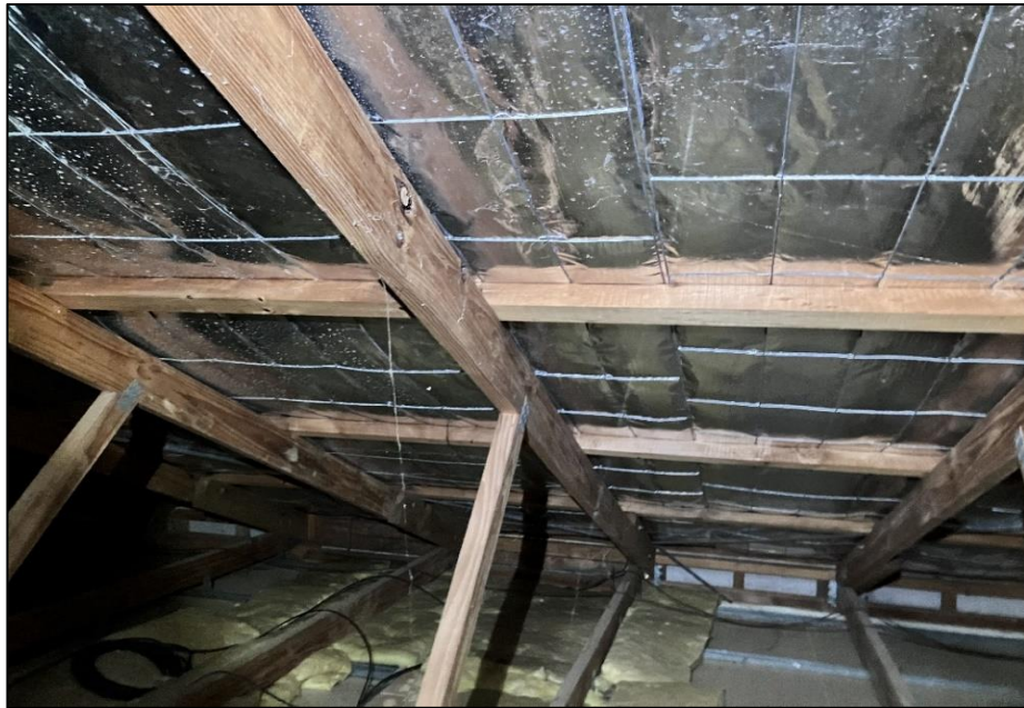
Photograph 9: B00C, rooms and areas in general, ceiling cavity, underside of roof, insulation, SMF identified visually.
