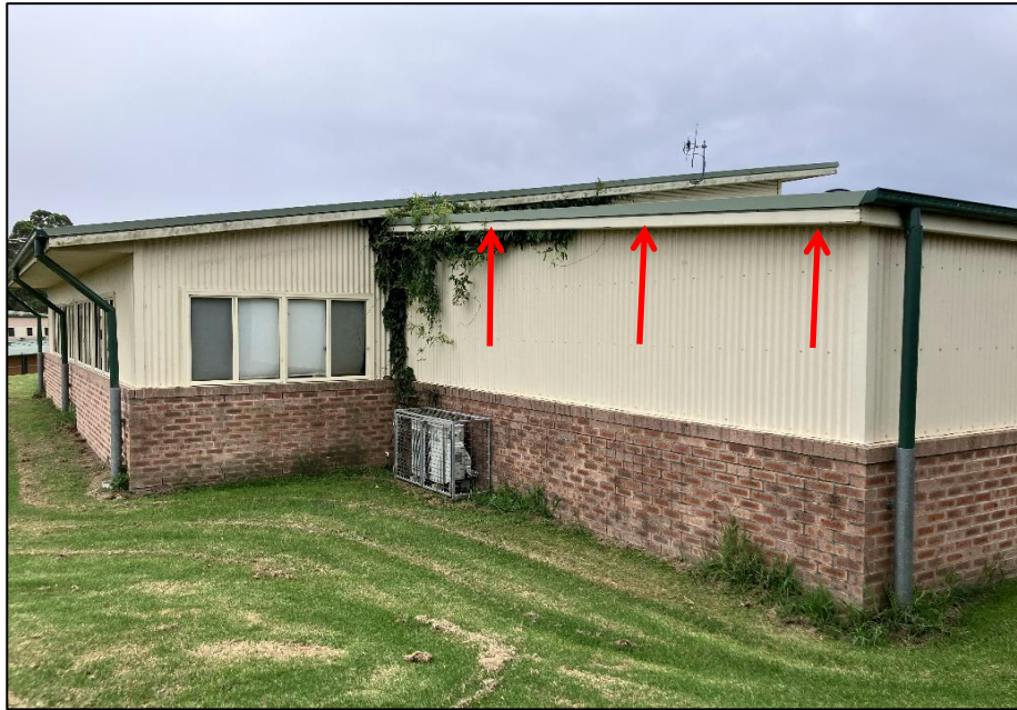
Photograph 1: B00V, exterior, western façade, south end, eave lining, no asbestos detected by analysis.
