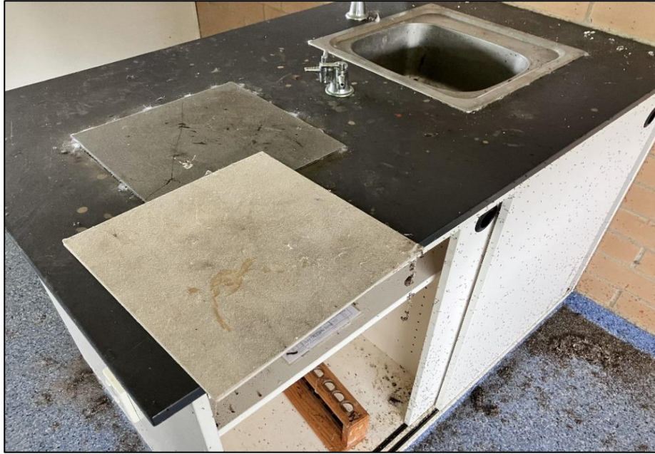
Photograph 5: B00C, interior generally, heat insulation pads generally, fibre cement product, suspected non-asbestos.
