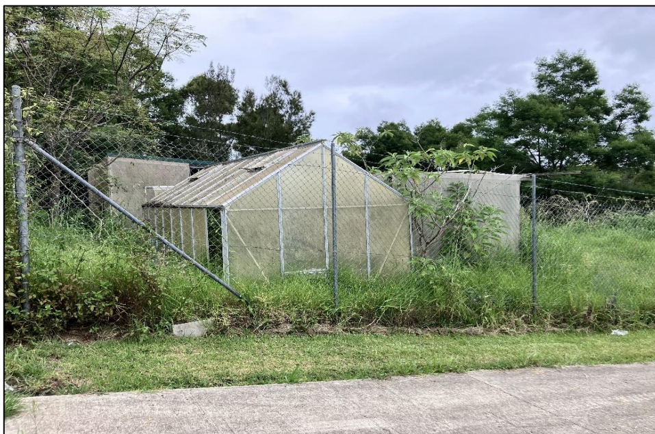
Photograph 3: B00F, inaccessible inside security (barbed wire) fencing.
