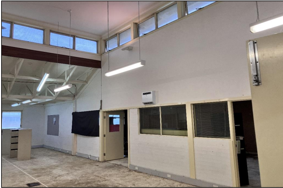
Photograph 7: B00B, BR0009, brick wall (white paint) and door frame (cream paint).
