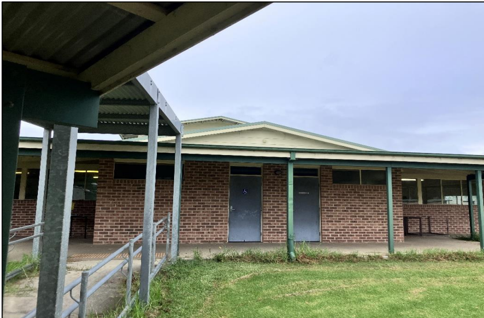
Photograph 2: B00A, exterior, upper level, wall and gables generally, weatherboard linings, suspected non-asbestos.
