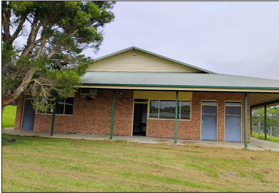
Photograph 1: B00E, exterior, north and south façade, gables, weatherboard linings, inaccessible.
