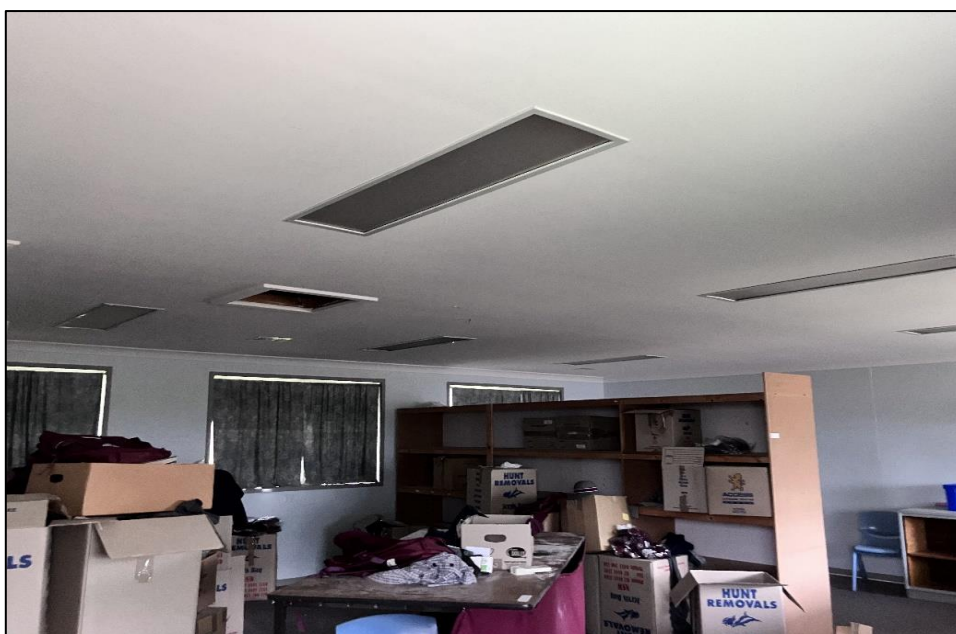
Photograph 4: B00T, rooms and areas in general, fluorescent light fittings, internal components, nil PCB (suspected).
