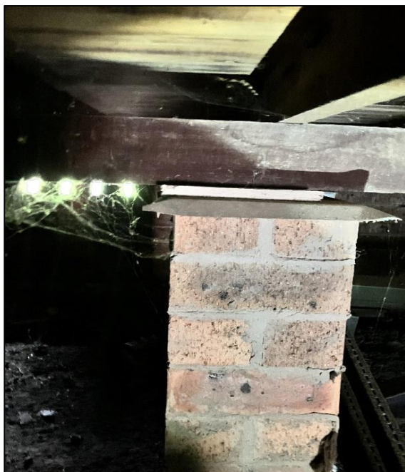
Photograph 3: B00P, sub-floor area, packing material, fibre cement sheeting, no asbestos detected by analysis.
