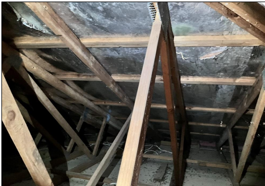
Photograph 14: B00W, ceiling cavity, underside of roof, insulation materials, SMF identified visually.
