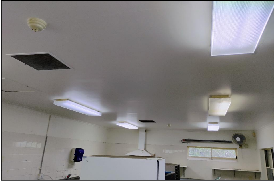
Photograph 3: B00U, interior, UR0002, ceiling, fibre cement sheeting, no asbestos detected by analysis.
