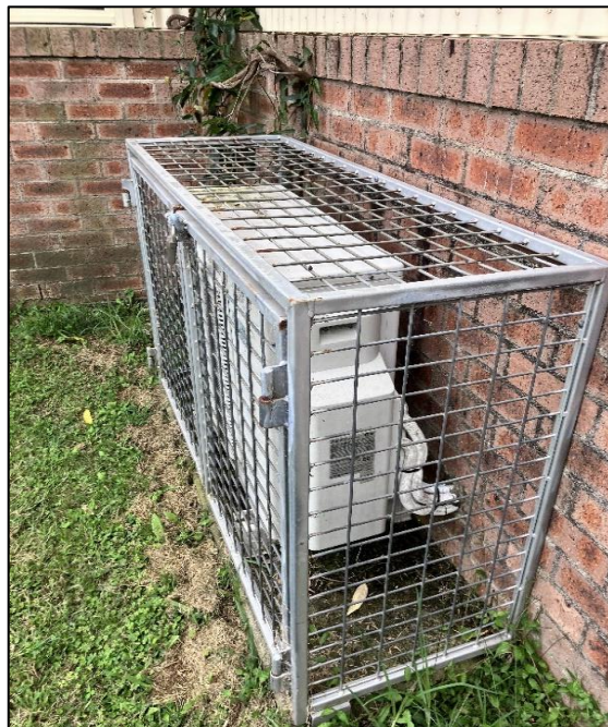
Photograph 8: B00V, exterior, western façade, south end, air conditioning unit, R410A, nil ODS identified.
