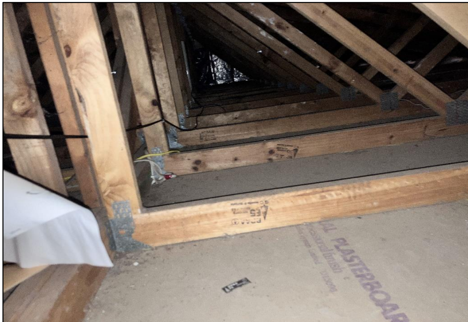
Photograph 4: B00S, interior, ceiling cavity, settled dust / debris, elevated lead concentration detected.
