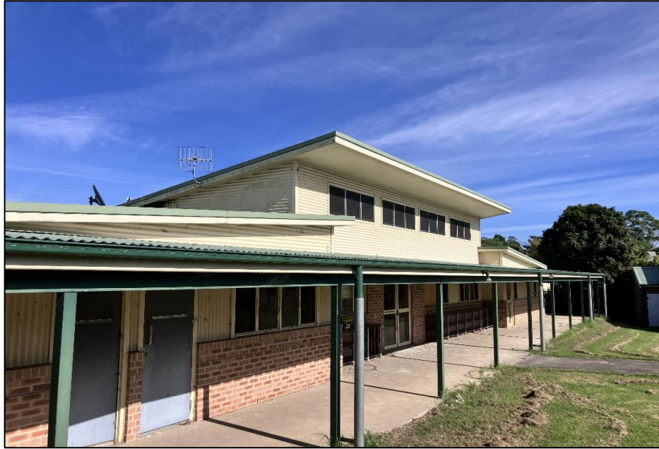
Photograph 5: B00V, exterior, east façade, timberwork (green and cream paints) and doors (grey paint).
