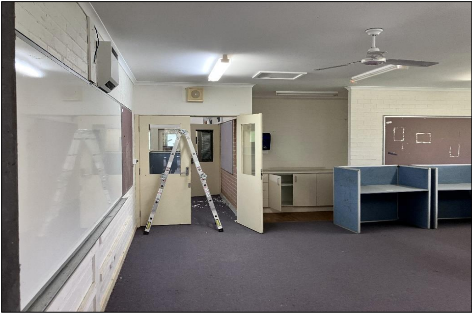
Photograph 12: B00A, rooms and areas in general, fluorescent light and fan fittings, internal components, nil PCB (suspected).
