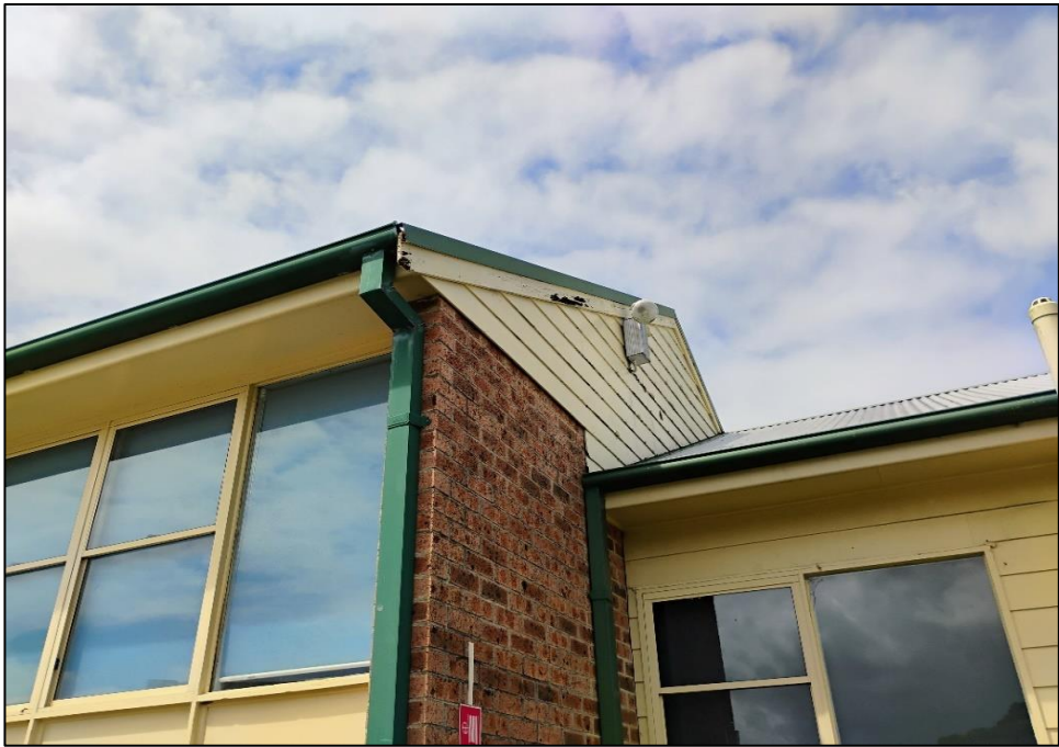
Photograph 2: B00Q, exterior, eave and gable lining, fibre cement sheeting, no asbestos detected by analysis.
