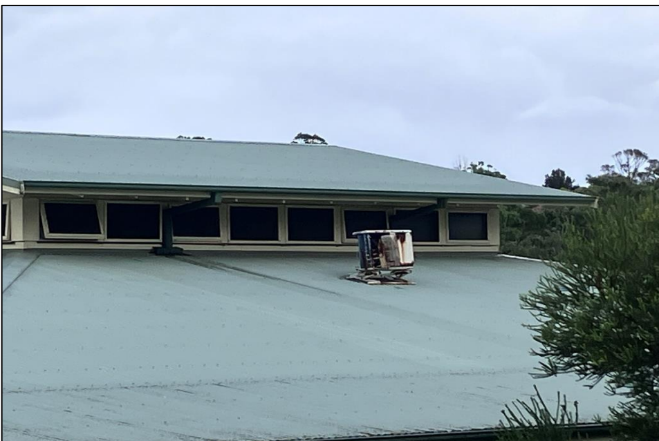
Photograph 13: B00A, exterior, roof, airconditioning unit(s), unidentified, inaccessible.
