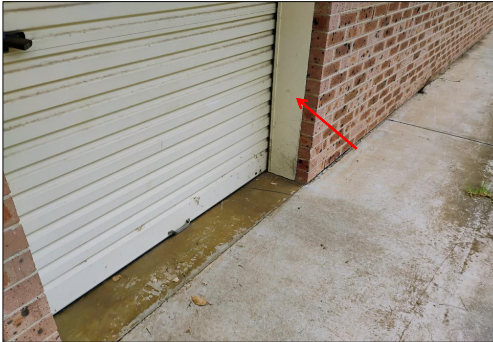
Photograph 3: B00D, exterior, framing around DR007 entrance, fibre cement sheeting, no asbestos detected by analysis.
