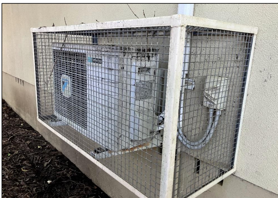
Photograph 18: B00W, exterior, northern façade, Daikin air conditioning unit, R410A, nil ODS identified.
