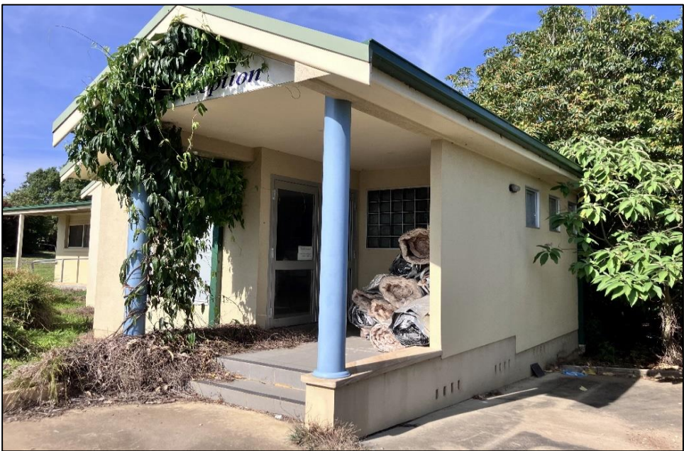
Photograph 12: B00W, WR0001, stored on porch area, rolls of insulation material, SMF identified visually.
