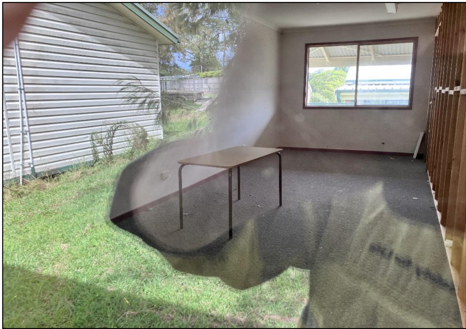
Photograph 4: B00R, interior, RR0003, materials in general, inaccessible (locked).
