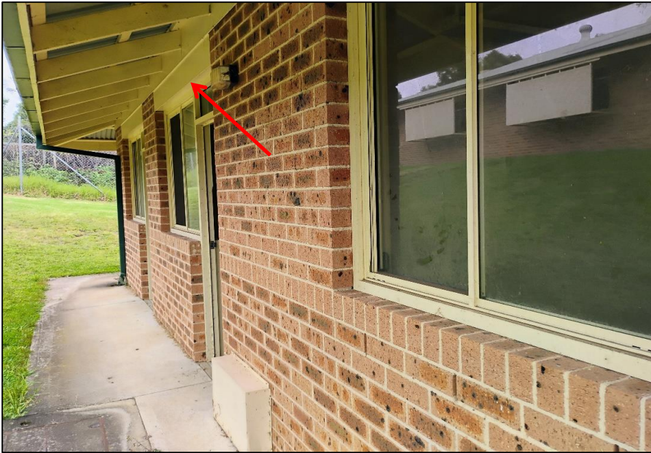
Photograph 3: B00E, exterior, typical wall, headlining, fibre cement sheeting, no asbestos detected by analysis.
