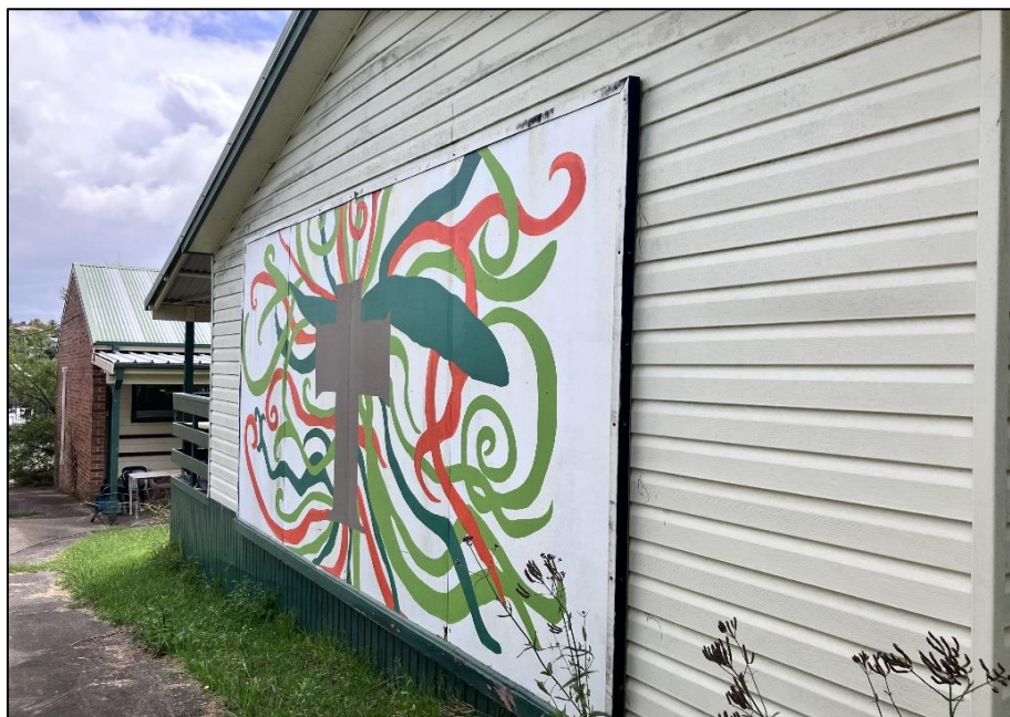
Photograph 2: B00R, exterior, southern façade, mural, fibre cement sheeting, no asbestos detected by analysis.
