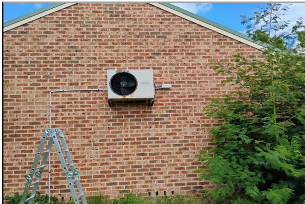
Photograph 2: B00P, exterior, northern façade, air conditioning unit, R22, ODS identified.
