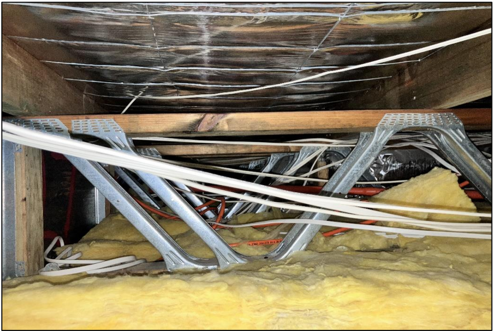
Photograph 4: B00H, rooms and areas in general, ceiling cavity, underside of roof, bulk insulation, SMF identified visually.
