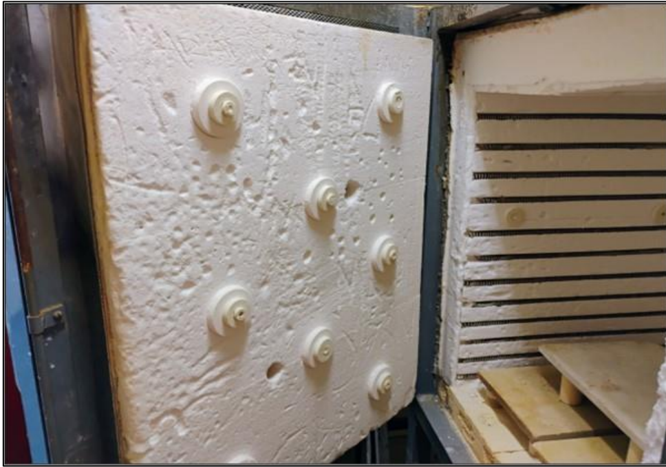
Photograph 7: B00E, interior, ER0016, pottery kiln, bulk insulation, no asbestos detected by analysis (SMF detected).
