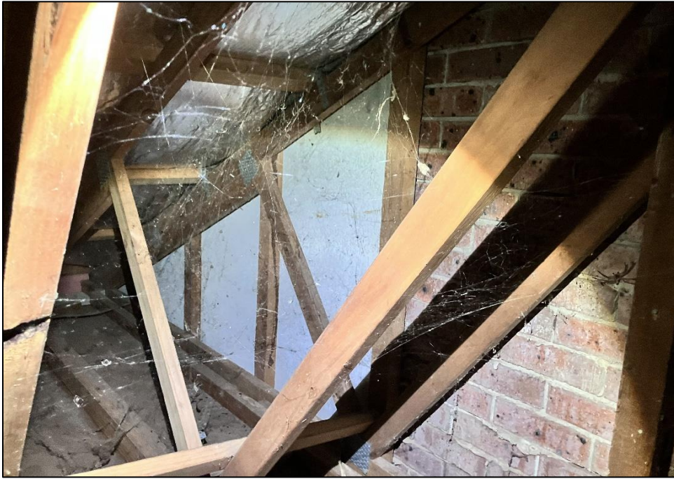
Photograph 3: B00Q, QR004, ceiling cavity, gable, fibre cement sheeting, no asbestos detected. Underside of roof, insulation, SMF identified.
