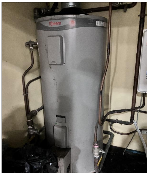
Photograph 6: B00I, interior, IR0013, hot water unit (circa 2001), bulk insulation, SMF (suspected).
