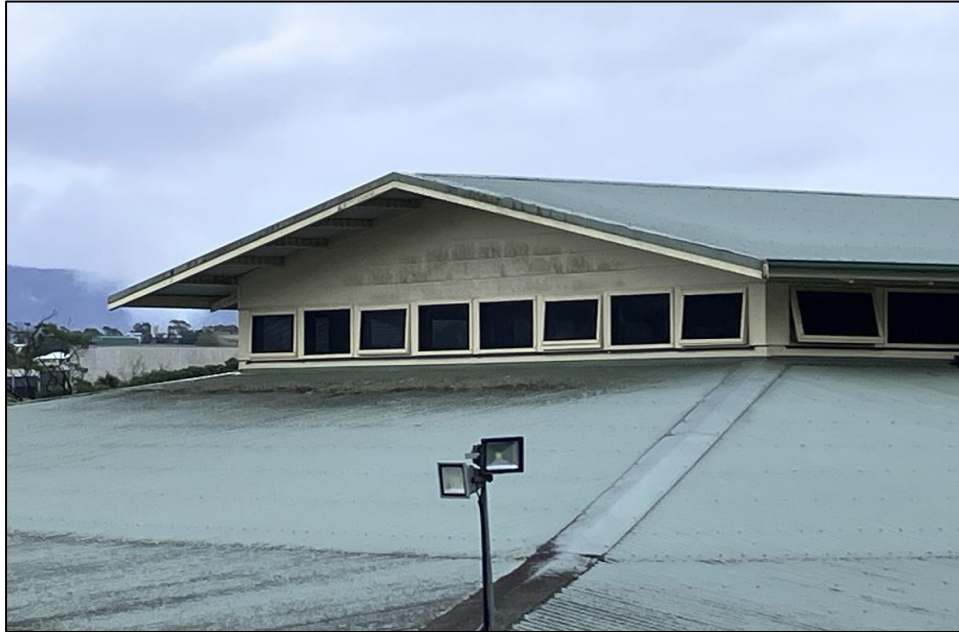
Photograph 1: B00A, exterior, upper level, wall and gables generally, weatherboard linings, suspected non-asbestos.
