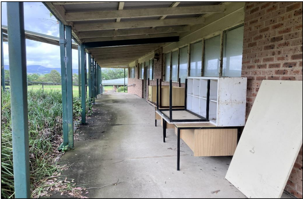
Photograph 2: B00B, exterior, lower level, walls generally, weatherboard linings, suspected non-asbestos.
