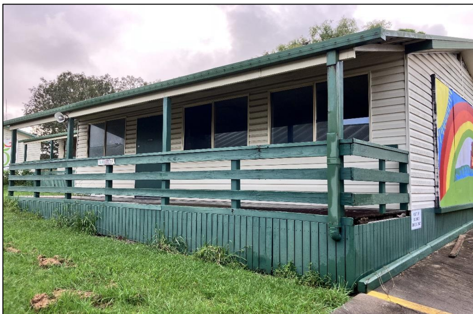
Photograph 3: B00T, exterior, west façade, timber deck and framework (green paint).
