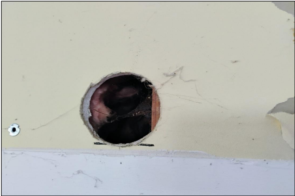
Photograph 6: B00D, rooms and areas in general, walls, insulation, SMF identified visually.
