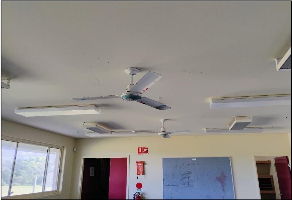
Photograph 12: B00E, rooms and areas in general, fluorescent light and fan fittings, internal components, nil PCB (suspected).
