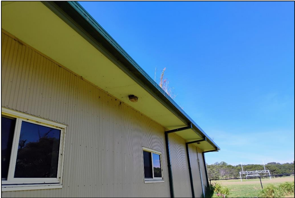
Photograph 3: B00H, exterior generally, eave linings, fibre cement sheeting, suspected non-asbestos.
