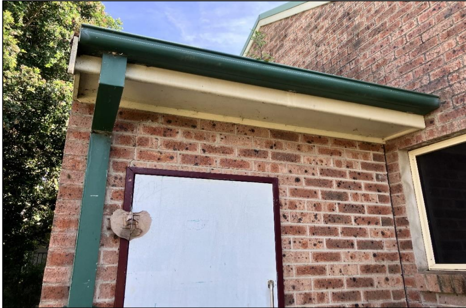
Photograph 1: B00W, exterior, WR0015, eave lining, fibre cement sheeting, no asbestos detected by analysis.
