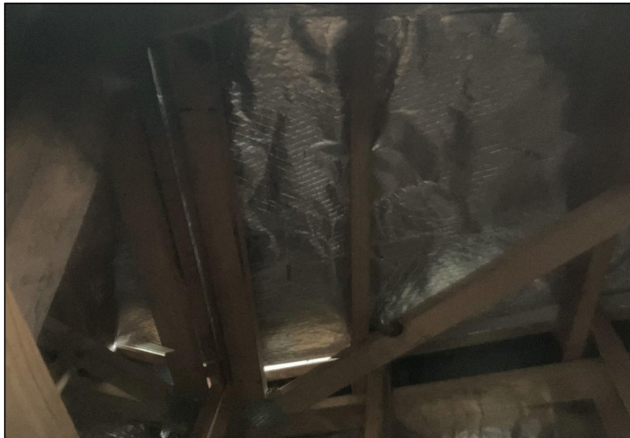
Photograph 5: B00S, interior, ceiling cavity, underside of roof, bulk insulation, SMF identified visually.
