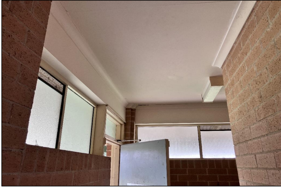
Photograph 5: B00A, AR0018 / 19, wall infill and ceiling linings, fibre cement sheeting, no asbestos suspected and/or detected by analysis.
