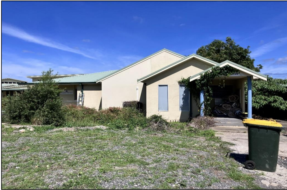
Photograph 5: B00W, exterior, northeastern façade, wall linings, fibre cement sheeting, suspected non-asbestos.
