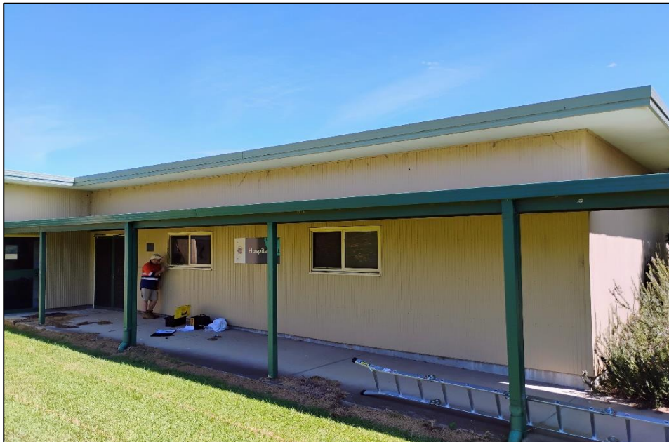
Photograph 2: B00H, exterior generally, eave linings, fibre cement sheeting, suspected non-asbestos.
