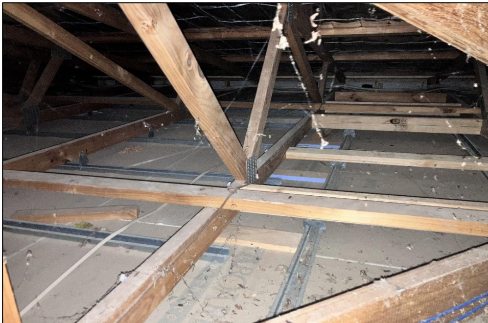
Photograph 8: B00B, ceiling cavity, settled dust / debris, elevated lead concentration detected.
