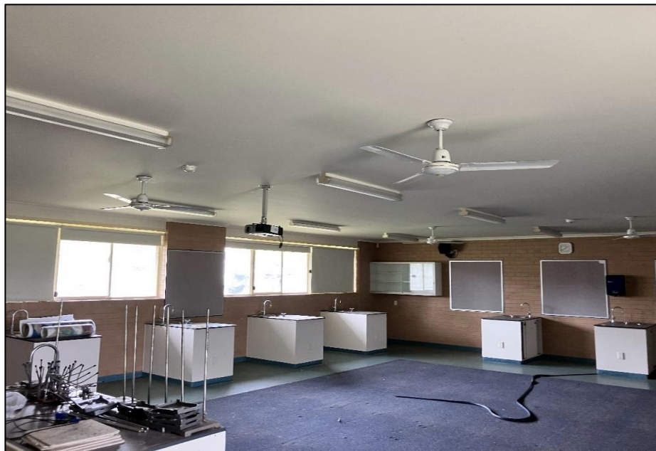
Photograph 10: B00C, rooms and areas in general, fluorescent light fittings and ceiling fans, internal components, nil PCB (suspected).
