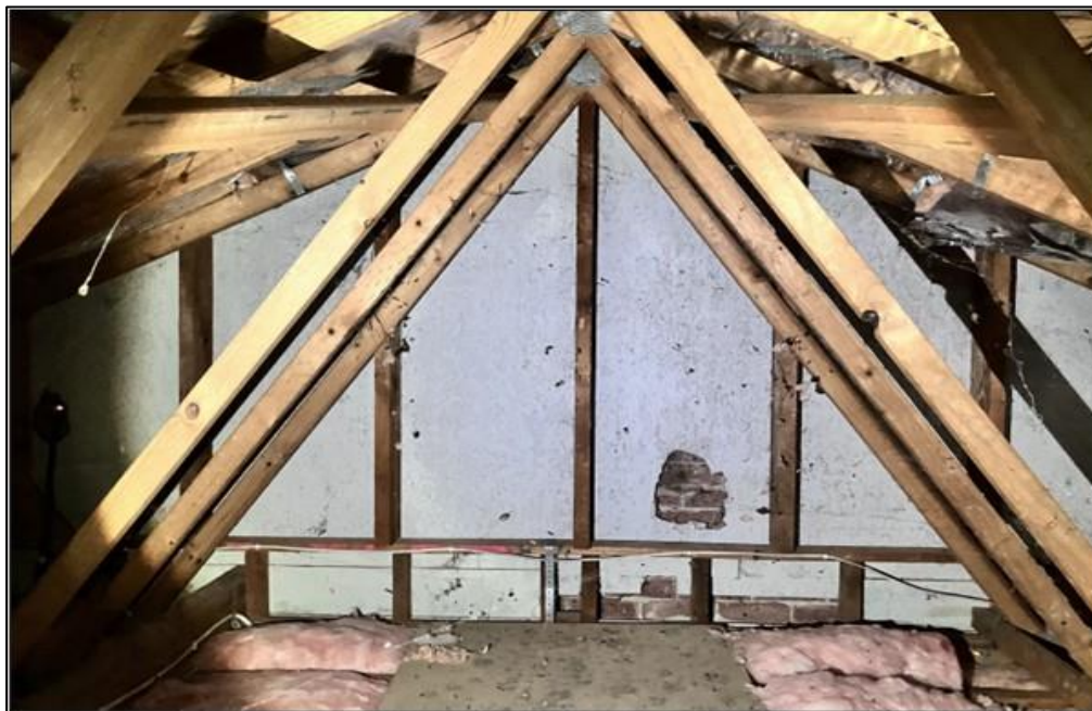
Photograph 6: B00P, ceiling cavity, gable, southern façade, fibre cement sheeting, no asbestos detected by analysis.
