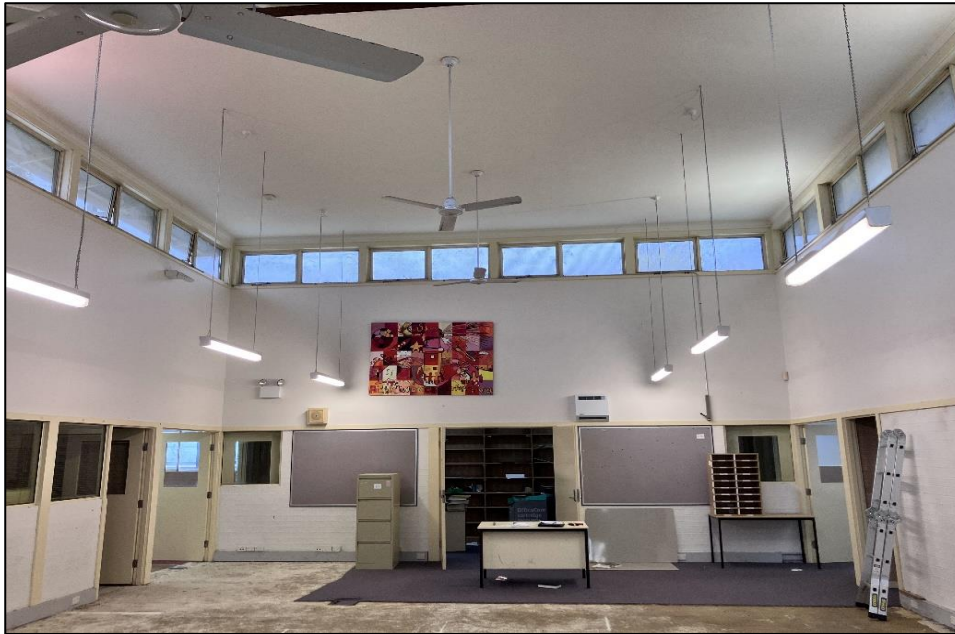
Photograph 5: B00B, BR0009, upper ceiling, suspected plaster product, suspected non-asbestos.
