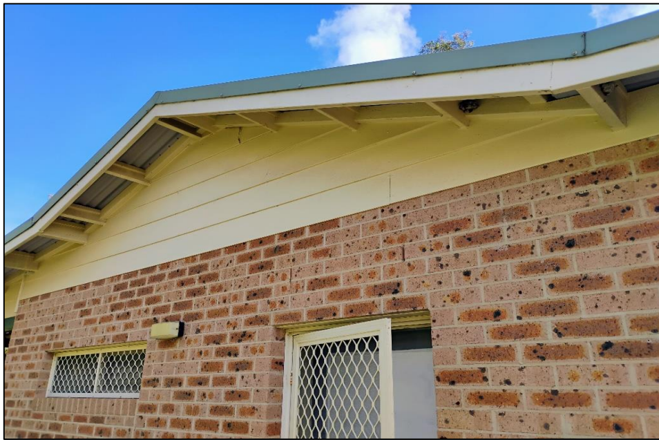
Photograph 1: B00U, exterior, northern façade, weatherboard lining, fibre cement sheeting, no asbestos detected by analysis.
