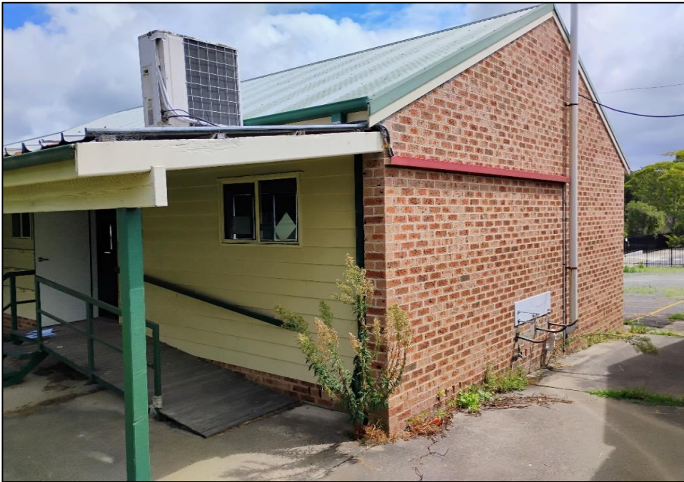
Photograph 8: B00Q, exterior,QR003, roof, air conditioning unit, R410A, nil ODS identified.
