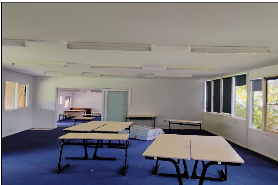
Photograph 10: B00P, rooms and areas in general, fluorescent light / fan fittings, internal components, nil PCB (suspected).
