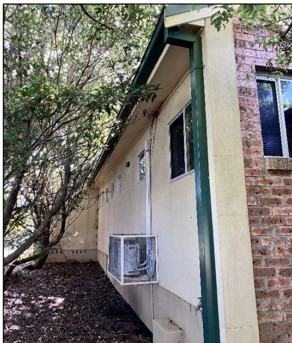
Photograph 4: B00W, exterior, northwestern façade, wall linings, fibre cement sheeting, no asbestos detected by analysis.
