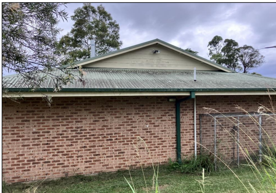
Photograph 1: B00C, exterior, gables, weatherboard linings, inaccessible.
