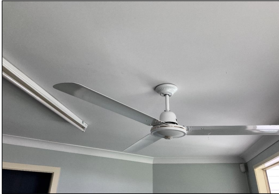
Photograph 7: B00S, rooms and areas in general, ceiling fans, internal components, nil PCB (suspected).
