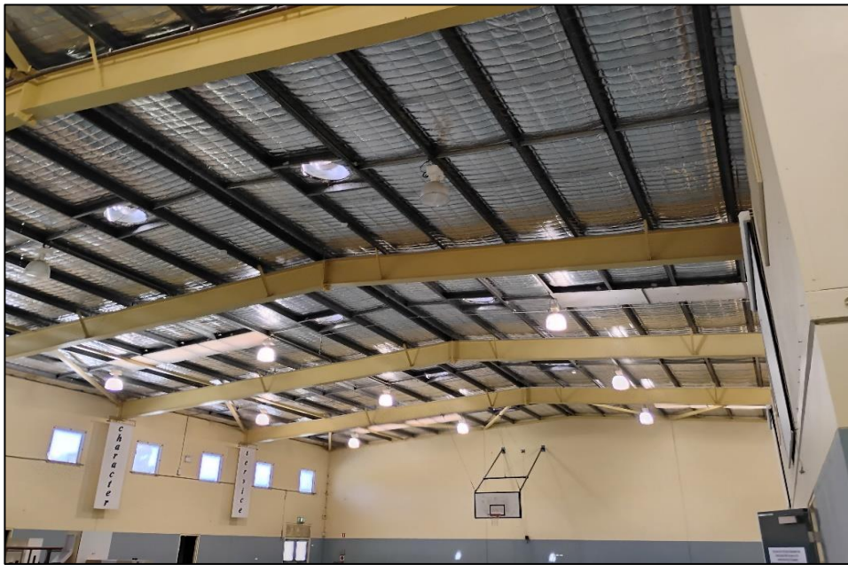
Photograph 7: B00I, interior, underside of roof, bulk insulation, SMF (suspected).
