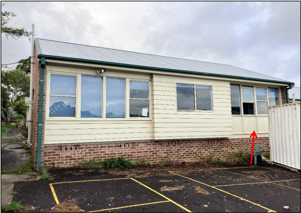
Photograph 1: B00Q, exterior, west façade, wall / infill panels, fibre cement sheeting, no asbestos detected by analysis.
