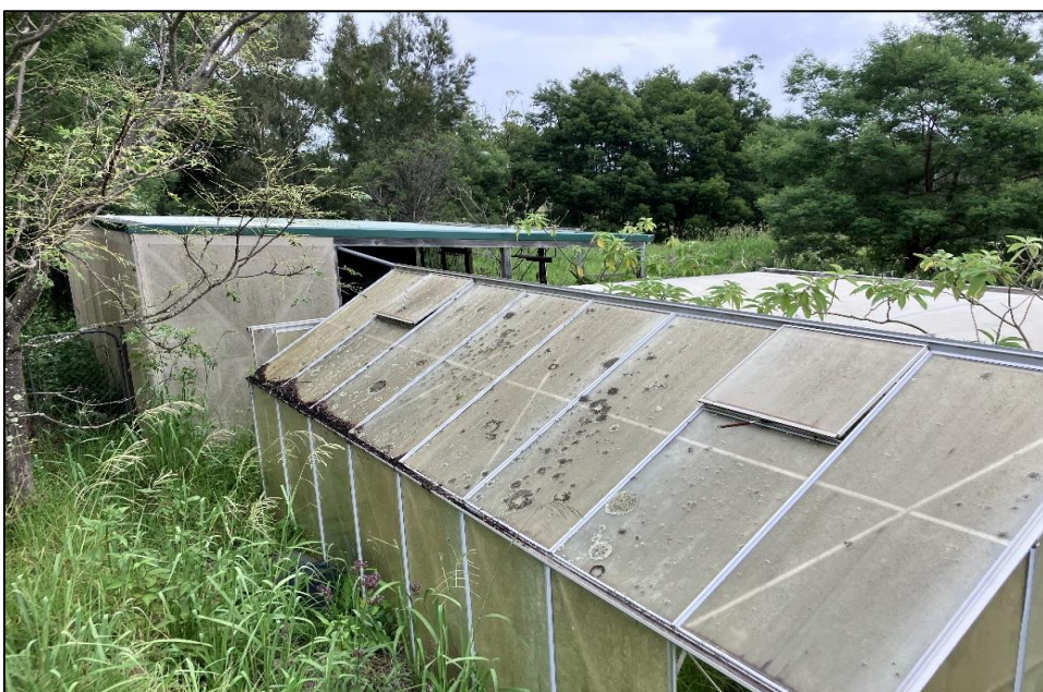
Photograph 4: B00F, view from top of ladder overlooking security fence.
