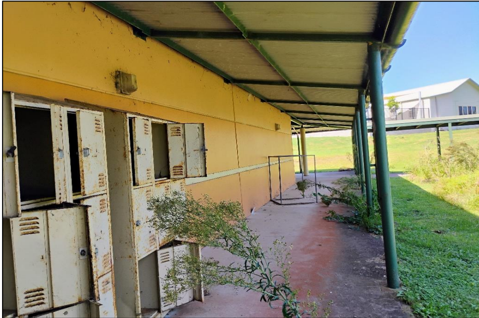
Photograph 3: B00I, exterior, southern façade, wall (orange paint) and awning support post (green paint).
