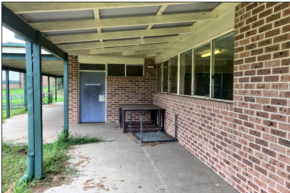
Photograph 8: B00A, exterior, north façade, timberwork, cream and green paints.
