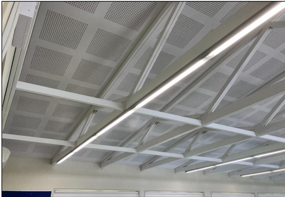
Photograph 6: B00V, interior, VR0004, ceiling, backing to perforated tiles, bulk insulation, SMF (suspected).
