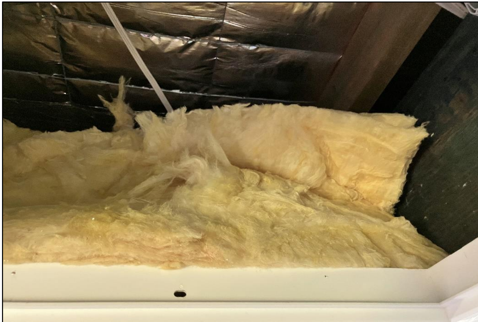
Photograph 5: B00H, rooms and areas in general, ceiling cavity, top of ceiling, bulk insulation, SMF identified visually.
