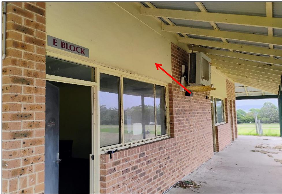
Photograph 2: B00E, exterior, north façade, infill, fibre cement sheeting, no asbestos detected by analysis.
