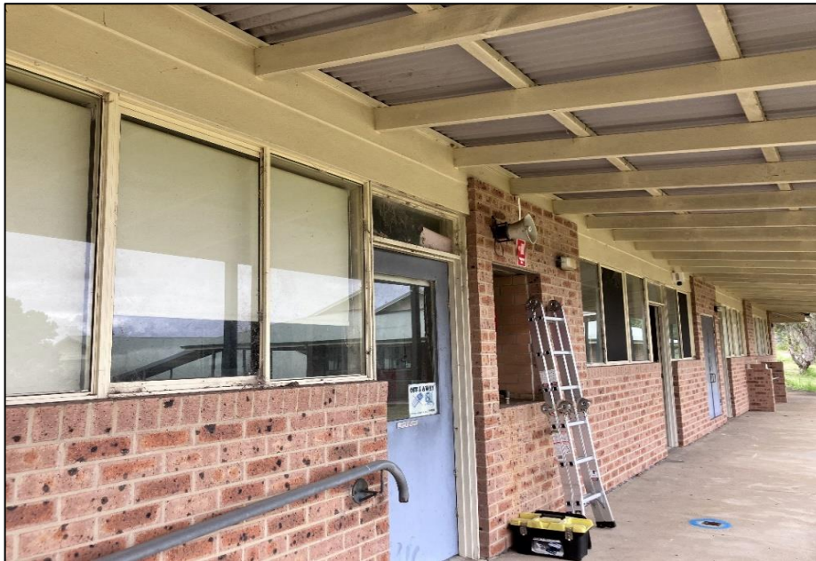
Photograph 6: B00C, exterior, ground level, western façade, door, grey paint.
