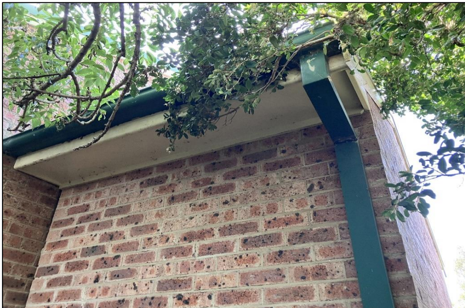
Photograph 2: B00W, exterior, WR0015, eave lining, fibre cement sheeting, no asbestos detected by analysis.
