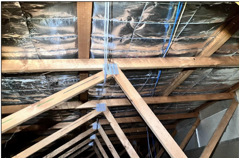
Photograph 9: B00B, rooms and areas in general, ceiling cavity, underside of roof, insulation, SMF identified visually.
