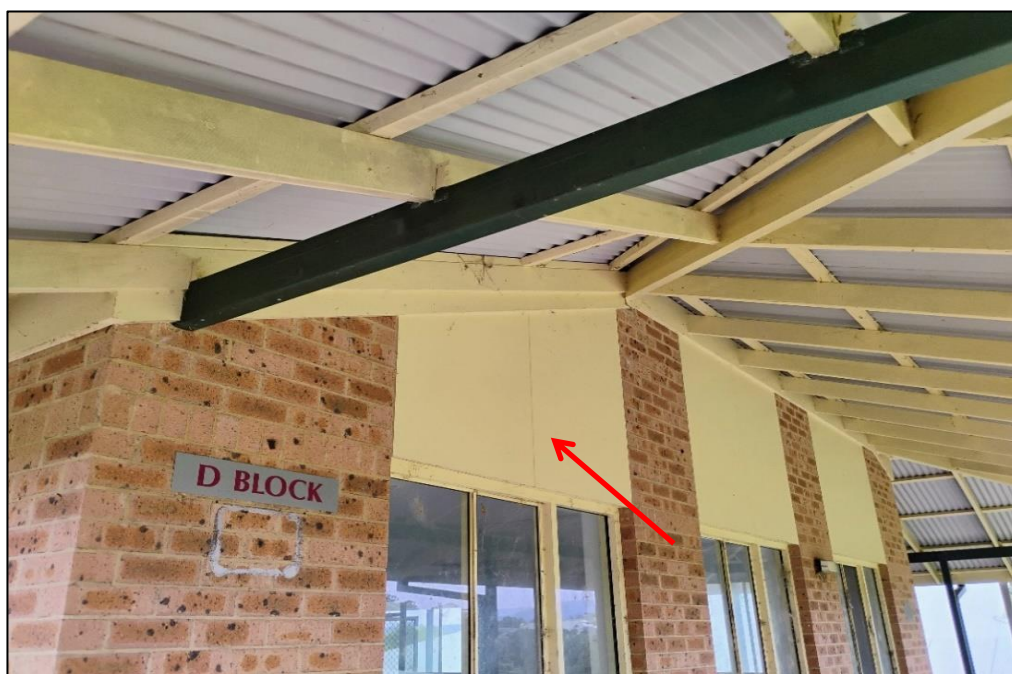
Photograph 2: B00D, exterior, north façade, infill, fibre cement sheeting, no asbestos detected by analysis.
